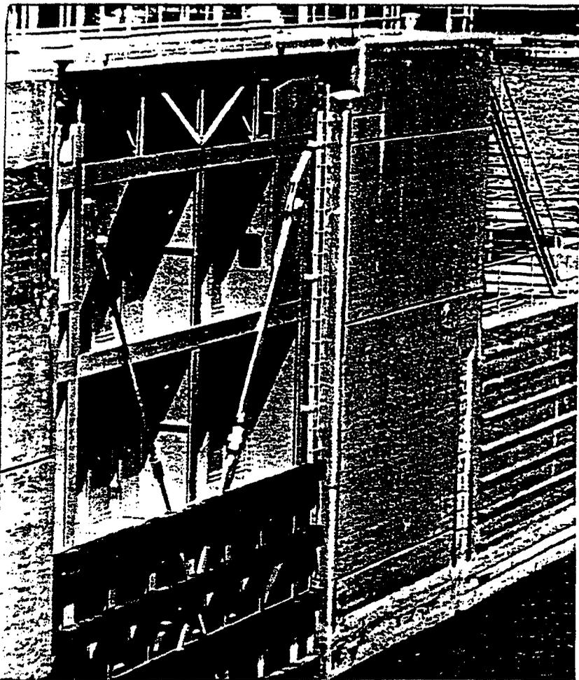
(b) Lower gate fully open and recessed in lock wall
